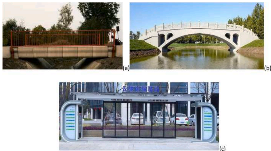
Fig. 1. 3D printed concrete bridges (a) constructed in the Netherlands with a span of 12.0 m [7], (b) built at the campus of Hebei University of Technology (China) with a span of 17.94 m [8], and (c) 3D-printed bus station [9].
