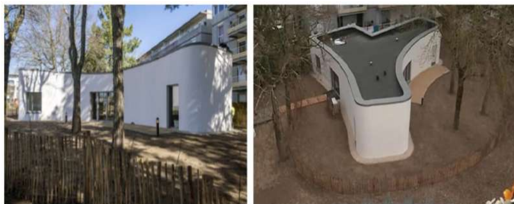
Figure 6. Yhnova™: A real-scale demonstrator of 3D printing with Batiprint™ [67].
