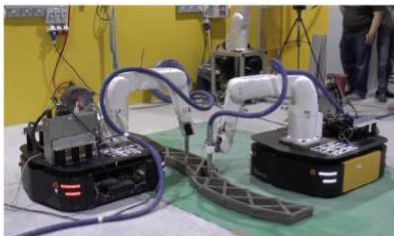
Figure 9. Concurrent printing of a large structure by two mobile robot printers [99].
