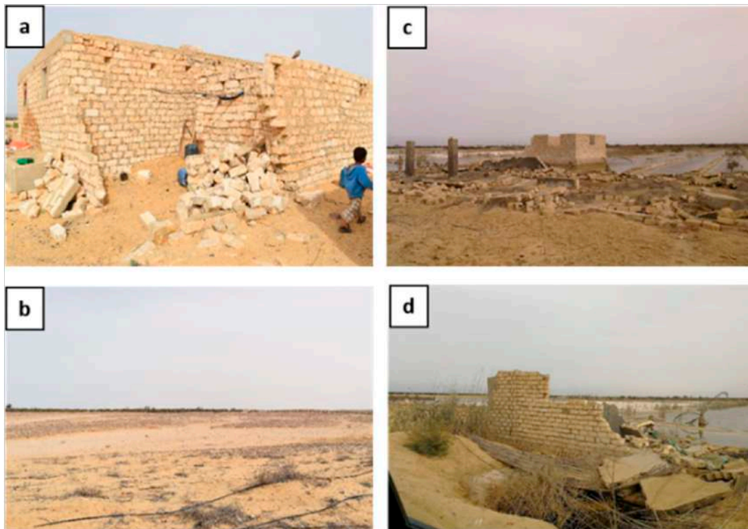
Figure 3. Consequences of a flash flood at Afouna Village: (a) damage to property, (b) one of the main flood stream paths in the village, (c) destruction of agricultural land, (d) wall collapsed in the main road.
