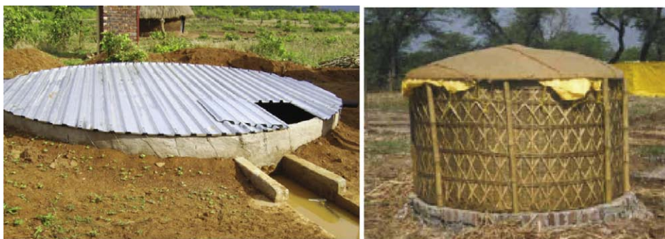
Fig. 3. Left: 30 m 3 RWH from ferrocement, underground (picture by Papenfus from [9]); right: bamboo tank developed by ARTI in Pune, India, uses a polythene sheet in a basket structure traditionally used for grain storage. Picture from [10].
