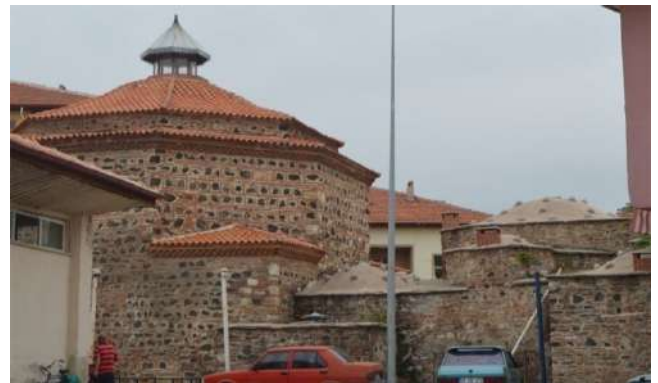
Figure 3. Wall braid in the Turkish bath with stone and brick material (Çinçin Hammam, Kula, Manisa, Turkey) [4]
