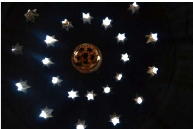
Figure 5. Elephant eyes on the dome of the warm space of Turkish bath (Osmanlı Hammam, Seferihisar, Izmir, Turkey) [4]
