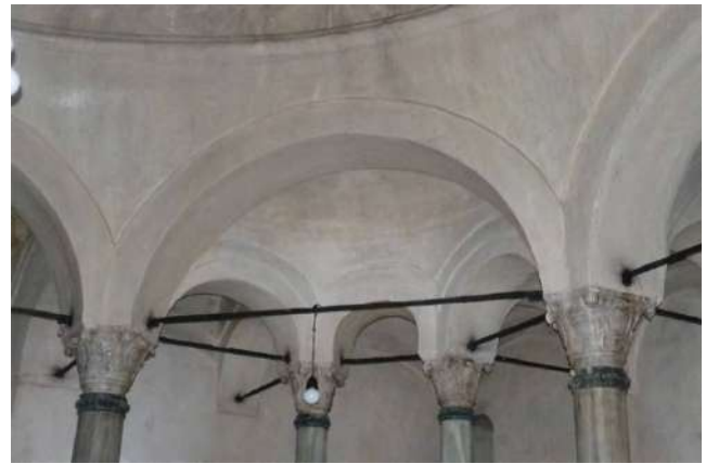
Figure 6. Marble columns in Turkish bath and arches connecting them (Cağaloğlu Hammam, Fatih, Istanbul, Turkey) [5]
