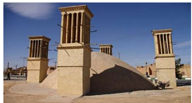
Figure 17. Ab anbar, featuring 4 badghirs, wind towers, Yazd, Iran
