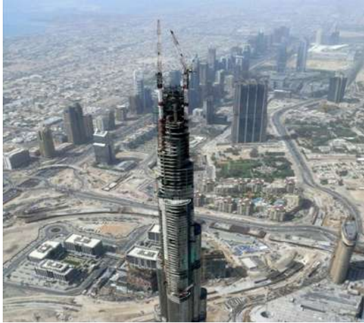
Figure 3. Burj Khalifa (Dubai) under construction
