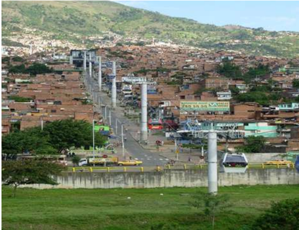
Figure 7. Metro-Cables, Medellin, Colombia
