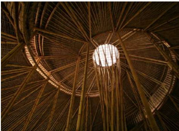
Figure 10. Bamboo Architecture, Ibuku Green School, Bali
