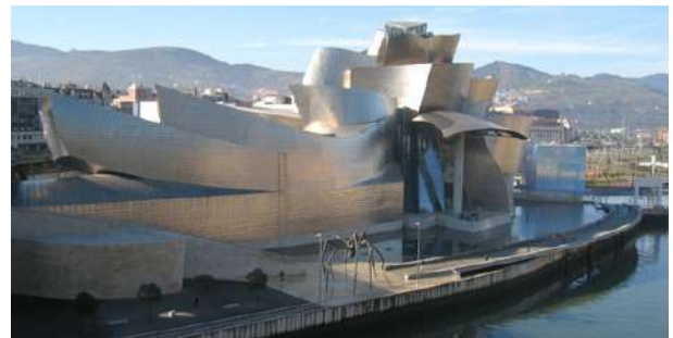
Figure 2. Guggenheim Museum Bilbao, Spain
