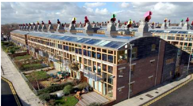
Figure 13. Zero Energy Development, Beddington, UK
